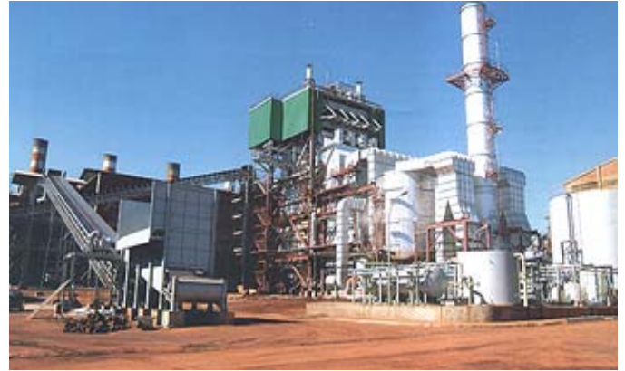
Figure 13: Santa Elisa plant
