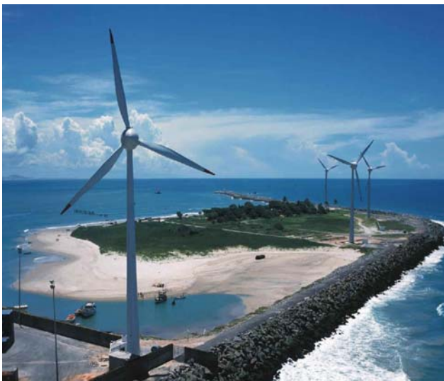
Figure 16: Mucuripe wind power plant
