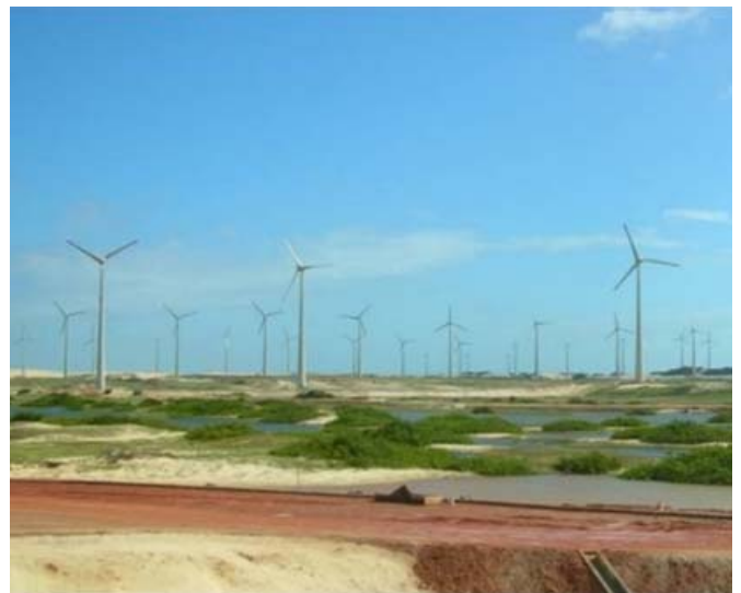
Figure 17: Rio do Fogo wind power plant
