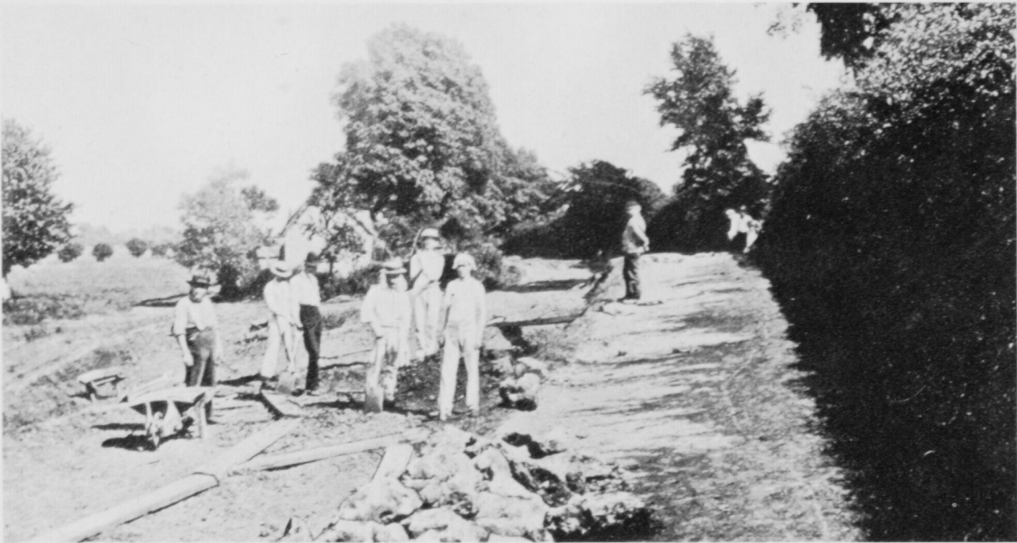
7 Building the Hinksey Road
