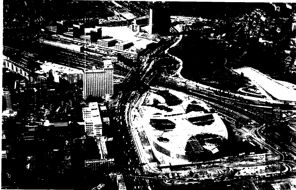
Aerial view of the Euralille project under construction, September 1994. Photo Daniel Rapaich.
