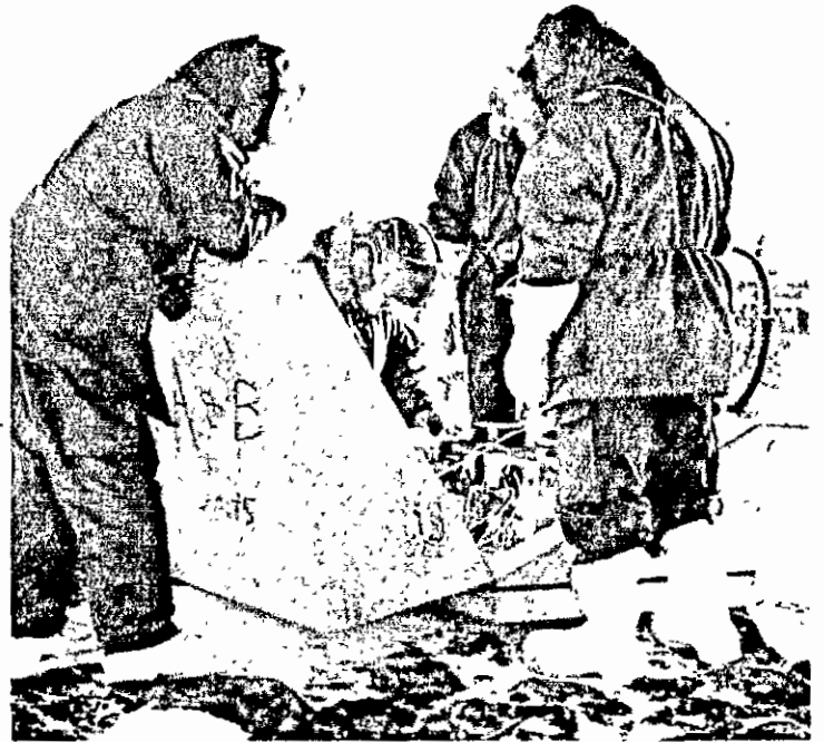
An insulated package containing the Microwave Ranging System transponding unit being installed atop a hill in one of the survey sectors. To operate properly, the transponders must have a clear line of sight between the unit and the aircraft.
