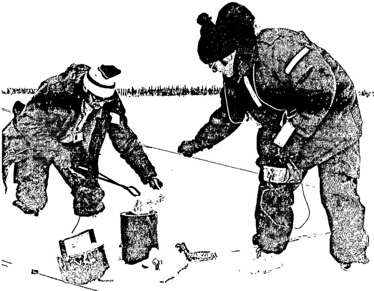
Radioactive debris being prepared for removal. In general, the materials were wrapped in plastic film to prevent dispersal of any dust or fine particles. The more radioactive objects were then manipulated into special shielded containers for safe transport.
